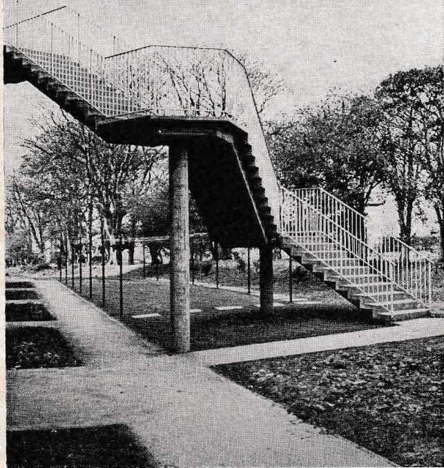
The heated staircase to the maisonettes
